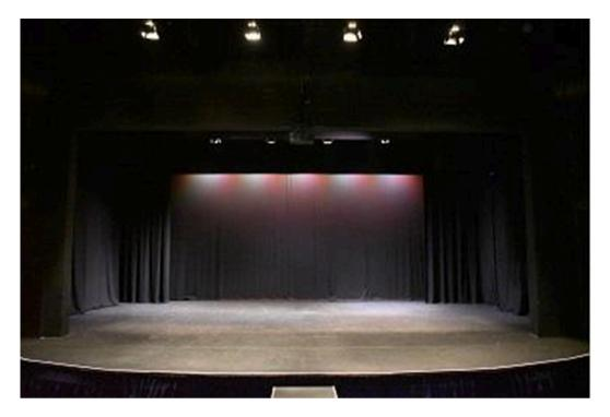
Slightly raked stage with a proscenium arch, and a single purchase counterweight fly system. Hardwood floor covered in Weathertex sheeting. Screwing into stage surface is permitted but must be authorised by centre staff.
