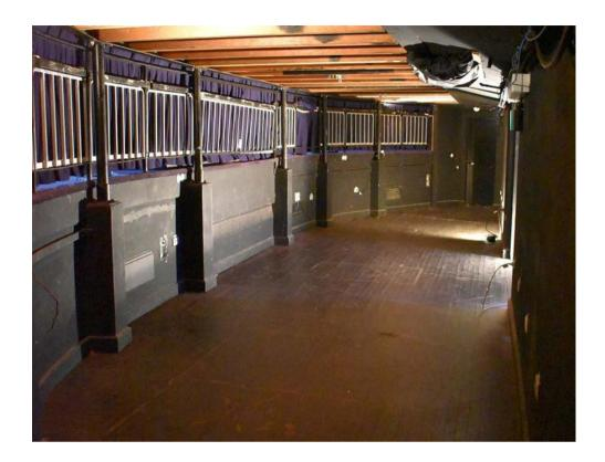
The orchestra pit is comprised of fixed floor sections that require three crew 1 hour to move. Dimensions  $10000 \times 3000 \times 2170$ mm (usable dimensions) Maximum capacity 35.
